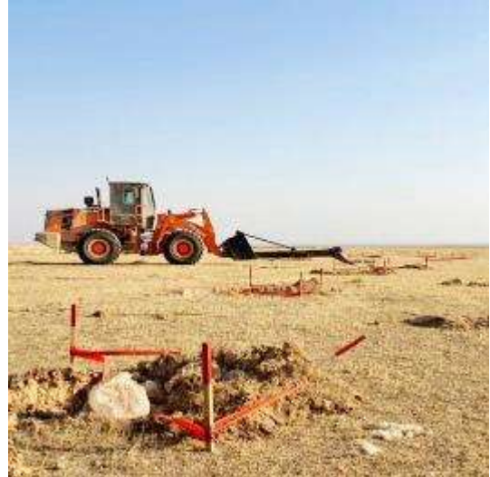
b) IED being lifted from the ground
