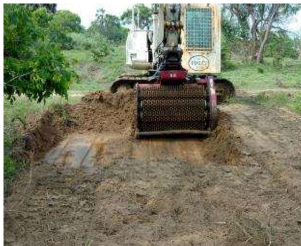
b) Follow up mechanical excavation and filtering
